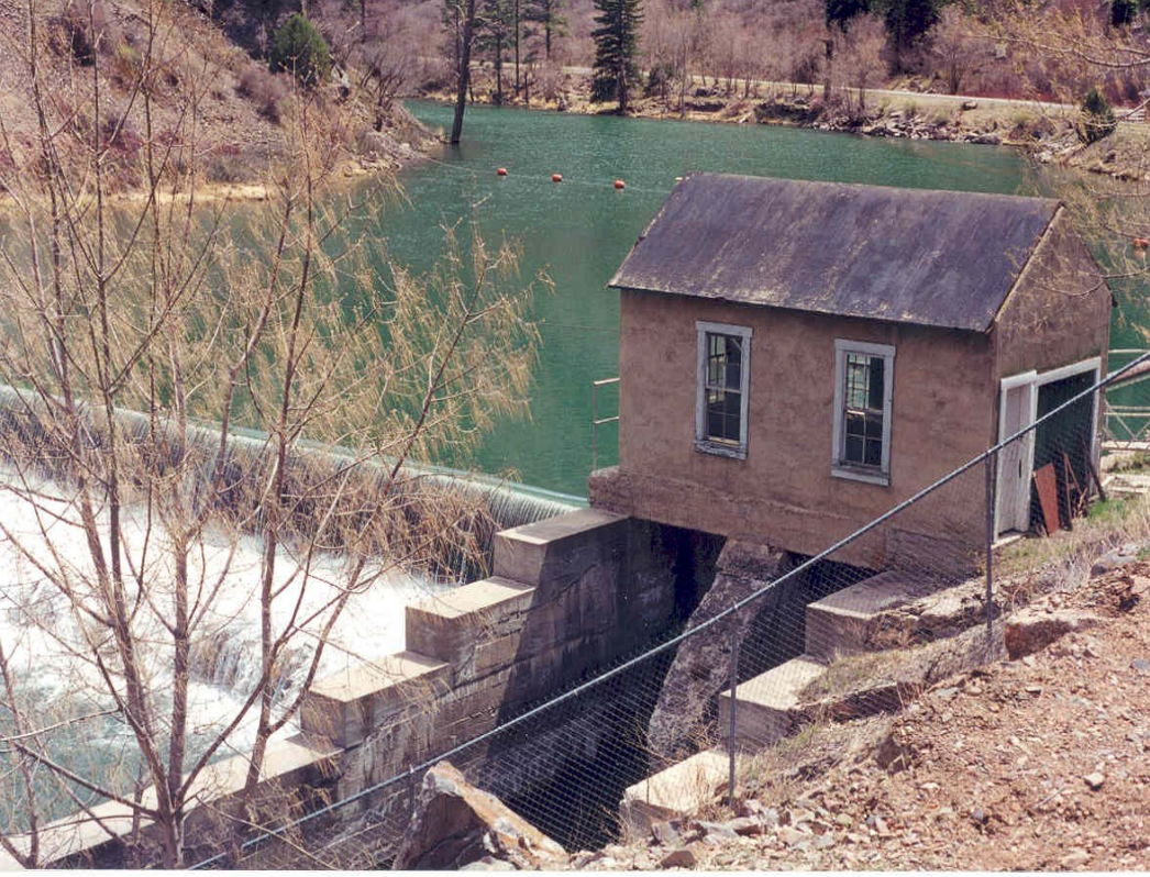
Gunnison Tunnel Diversion Dam and Intake
