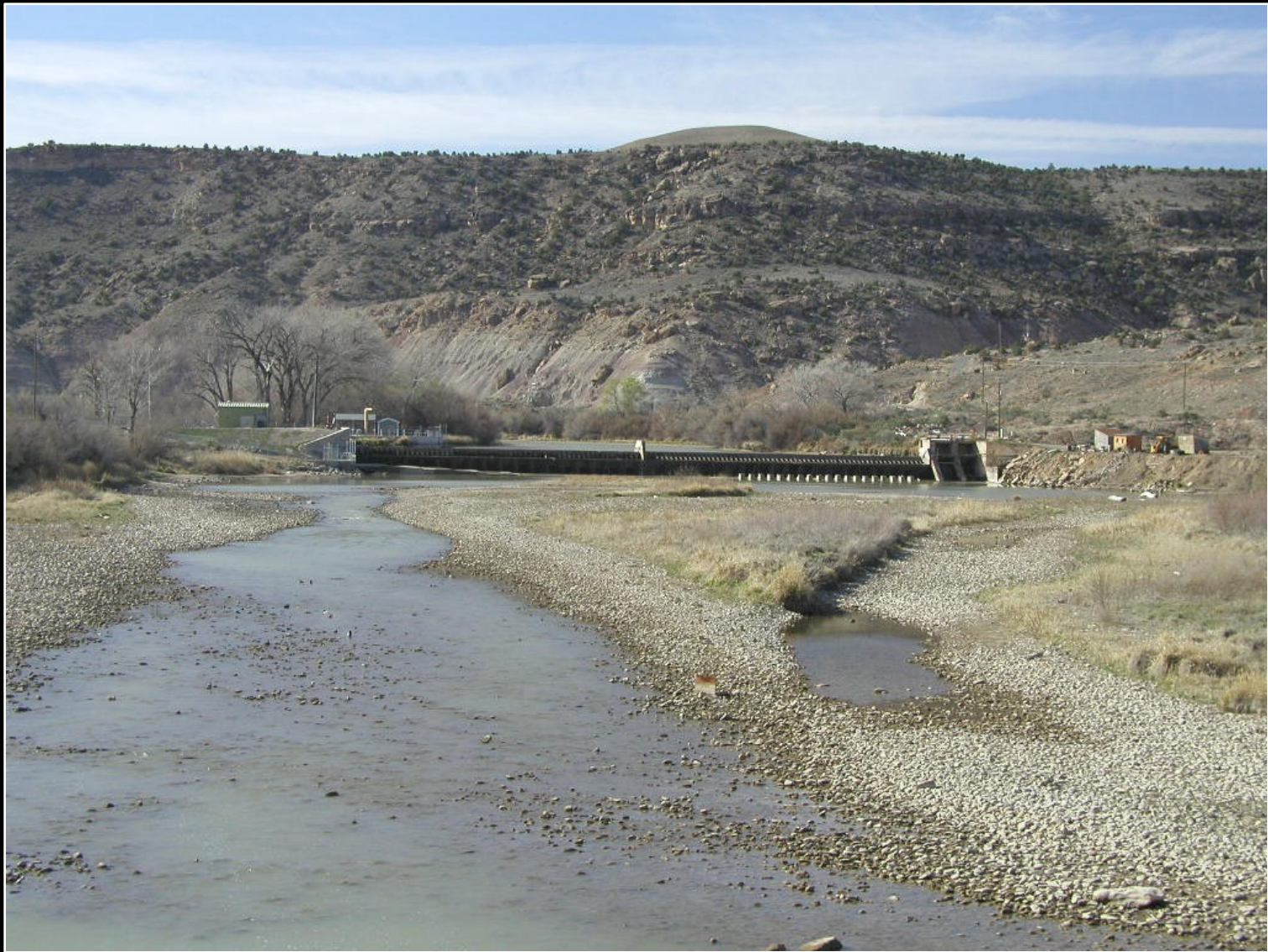
Redlands Dam; looking upstream, low flow conditions
